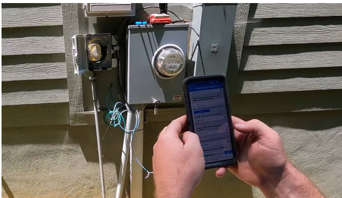
Premises Installation Projects
